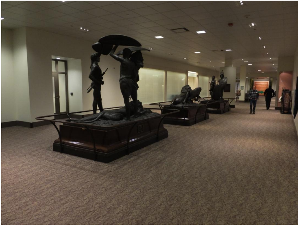
Figure 45-- Railings Not Cane Detectable on Ground Level Central Corridor
