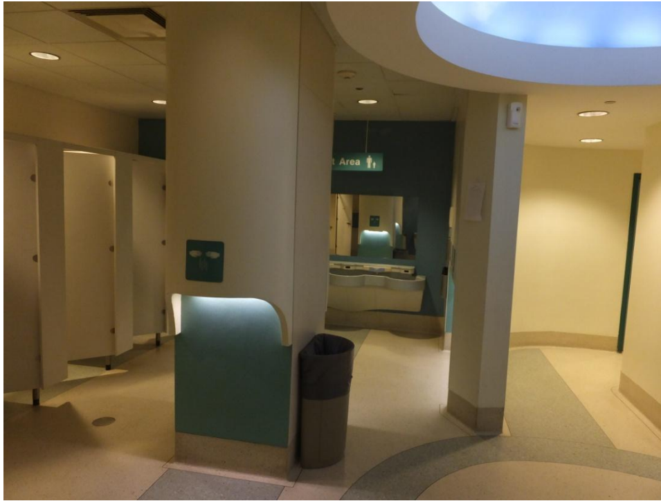
Figure 59 -- The Lower Level Men's Restroom at West Entry has Hand Dryer that is not Cane Detectable
