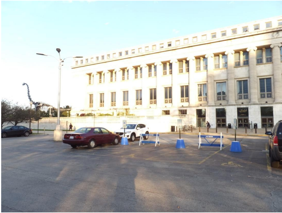
Figure 42 - Designated Accessible Parking and Approach to Accessible West Museum Entrance
